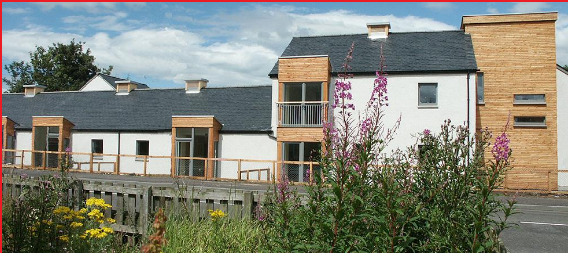
Fairfield Housing Cooperative, Perth , Scotland
