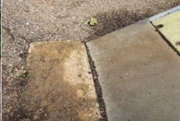
**Finding:** The kicker plate has sunk more than 5mm below the surrounding surface level, BS EN 14974 recommends a in level maximum of 5mm with 3mm preferred
