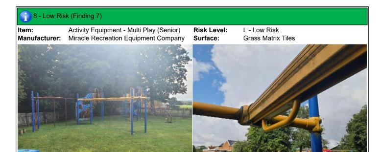
Finding: There are no buffers fitted to the mono rail Action: Provide buffers
