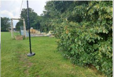
Finding: The overhanging foliage forms a hard object within Action: Cut back and maintain a 2m falling space the falling space of the equipment in contravention of the requirements of BS EN 1176 Part 1
