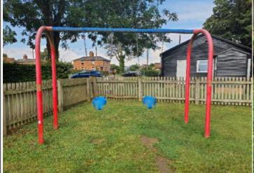
**Finding:** The connecting links are in excess of 8.6mm and less than 12mm and fail the requirements of BS EN 1176 Part 1; clause 4.2.13, Chains
