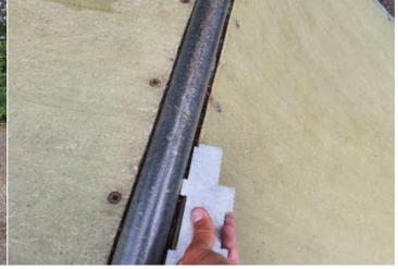
**Finding:** Joints between the riding surfaces should not be **Action:** Take corrective action to ensure that the gaps greater than 5mm to meet the requirements of BS EN 14974 between the joints do not exceed 5mm
