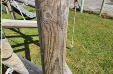
**Finding:** There are a number of redundant staples attached **Action:** Remove redundant staples to the equipment
