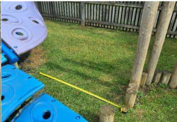
Finding: The log walk forms a hard object within the falling Action: Monitor - No remedial work recommended space of the equipment in contravention of the requirements of BS EN 1176 Part 1
