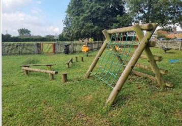
**Finding:** There is some strimmer / machinery damage apparent on the posts, this can penetrate the preservative applied to the timber and accelerate the rotting process
