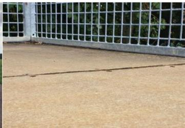
**Finding:** There is a change in the level of the rolling surface **Action:** Monitor - No remedial work recommended in excess of 3mm and the item fails the requirements of BS
