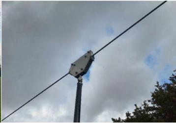
Finding: The nylon inserts are worn or missing at the point Action: Replace worn or missing inserts as required the cable enters the traveller
