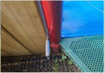
**Finding:** There is/are finger entrapment/s in the slide starting section and the item fails to meet the requirements of BS EN 1176 Part 1 4.2.7.6 Entrapment of fingers
