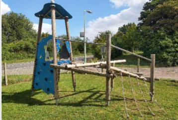
**Finding:** There is/are finger entrapment/s in the climbing wall and the item fails to meet the requirements of BS EN 1176 Part 1 4.2.7.6 Entrapment of fingers
