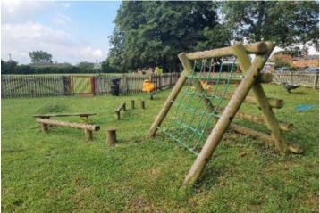
**Finding:** The timber stepping post forms a hard object within the falling space of the A frame climber in contravention of the requirements of BS EN 1176 Part 1
