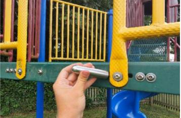
Finding: There is/are finger entrapment/s in the frame and Action: Monitor - No remedial work recommended the item fails to meet the requirements of BS EN 1176 Part 1
