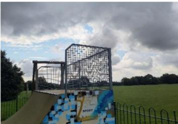
**Finding:** The height of the barrier is less than 1200mm and **Action:** Monitor - No remedial work recommended fails the requirements of BS EN 14974
