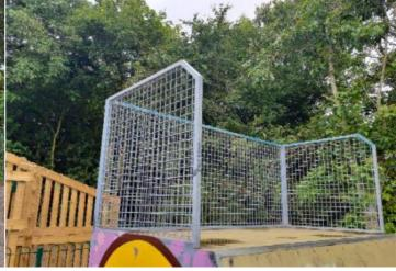
Finding: The height of the barrier is less than 1200mm and Action: Monitor - No remedial work recommended fails the requirements of BS EN 14974
