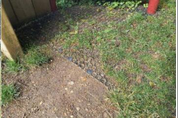
**Finding:** The edges of the grass mat surface have not been **Action:** Tuck in edges of grass mat to remove trip hazards installed in accordance with the API Code of Practice
