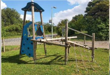
Finding: The ropes/nets are worn/damaged in places
