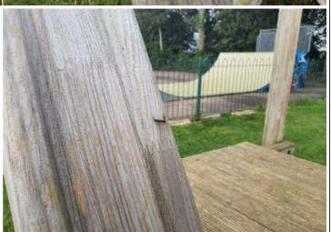
**Finding:** There are a number of redundant staples attached **Action:** Remove redundant staples to the equipment
