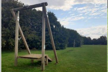
**Finding:** The seat connection cannot be inspected without dismantling the seat
