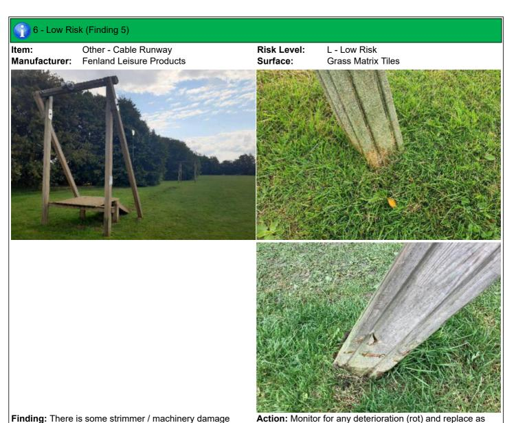
**Finding:** There is some strimmer / machinery damage apparent on the posts, this can penetrate the preservative applied to the timber and accelerate the rotting process
